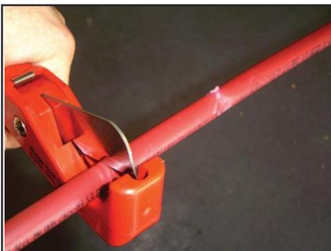
Inspect all tubing and fittings before and after installation. Cut out and replace all damaged sections or fittings.
