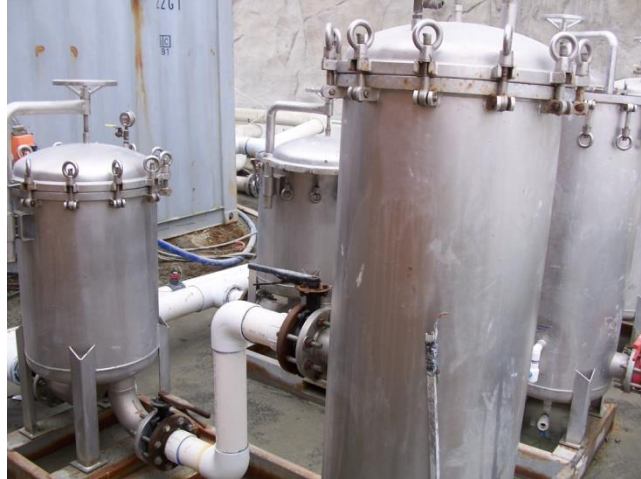
Figure C-3. Bag/Cartridge Filters
