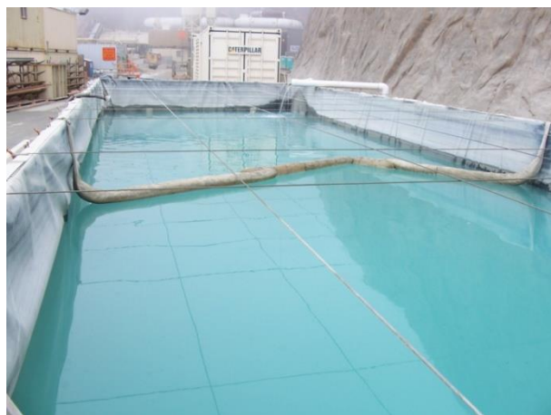
Figure C-2. Sedimentation Tank
