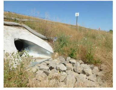
**Outlet Protection/Velocity Dissipation Devices** What is the BMP called? \_\_\_\_ What BMP objectives does it address? Soil Stabilization Sediment Control
