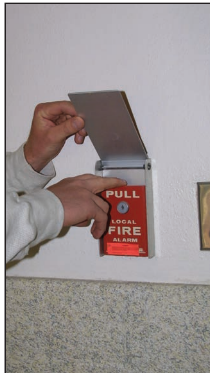
Figure 14.41 A double-action pull station has a panel that must be lifted so the operator can access and operate the pull station.
