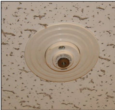
Figure 14.21 Heat detectors set to predetermined temperature ratings should be installed in ceilings in areas that are expected to accumulate heat.
