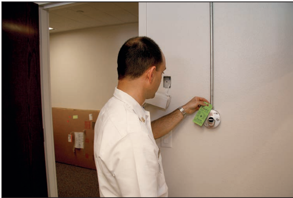
Figure 14.46 Check that inspection records are up-to-date.
