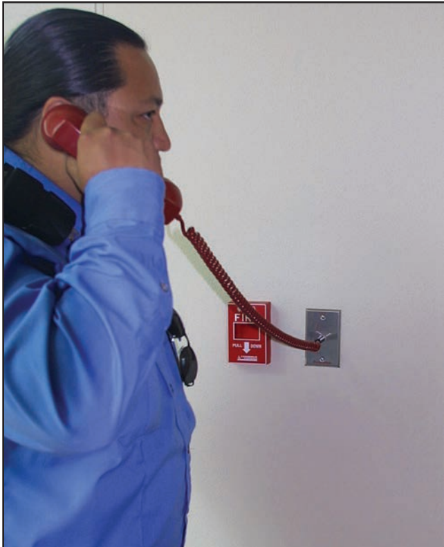
Figure 14.18 An intercom or other two-way system may be used when it is necessary for occupants to respond to officials giving them instructions during an emergency.
