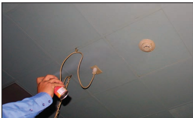
Figure 14.45 It is important to use approved testing procedures for smoke heat detectors.
