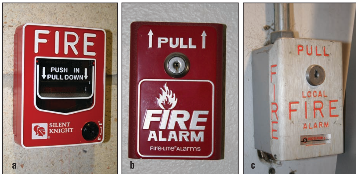
Figures 14.39 a-c Manually operated alarm-initiating devices may look slightly different, but all are important tools for signaling emergencies.
