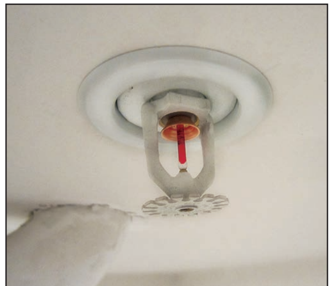
Figure 14.23 Frangible bulb detectors are designed to activate when the glass bulb breaks in response to heat.
