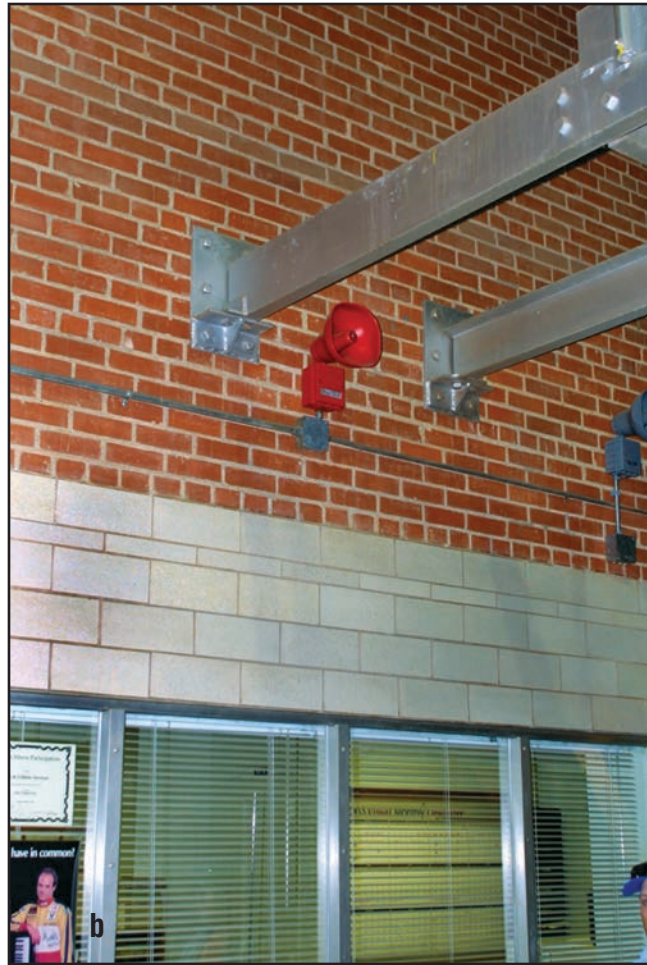
Figures 14.7 a-c Notification devices include bells, horns, strobe lights, and speakers.
