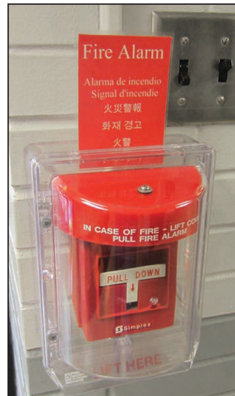
Figure 14.42 A manual alarm may require a cover to prevent damage. Courtesy of Rich Mahaney.
