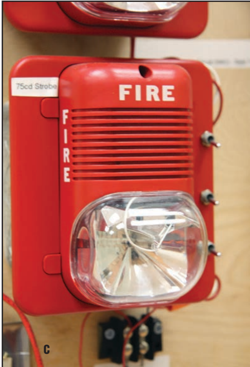
Figures 14.7 a-c Notification devices include bells, horns, strobe lights, and speakers.
