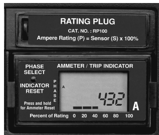
Combination Local Current Meter and Trip Indicator
