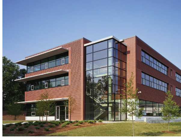
Figure 4.7. Building exterior with light shelves.
