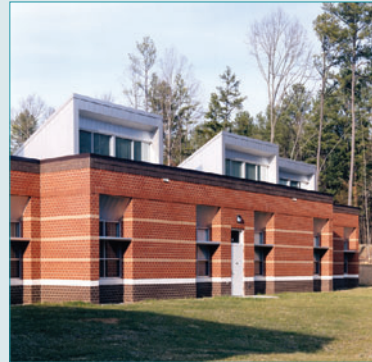
Figure S4.2 South-facing monitors.
