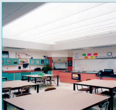
Figure S4.3. Classroom daylight monitors.
