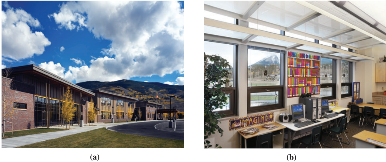
Figure 4.22. (a) Silverthorne Elementary School exterior and (b) classroom lighting system.
