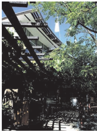
Figure 4-8. (a) The entry elevation of Real Goods Solar Living Center makes use of overhangs, a recycled-redwood trellis, and adjustable awnings. (b) The interior reveals its curving, stepped roof, east-facing clerestory windows, and light shelves that deliver natural light deeper into the interior without overheating or glare.
