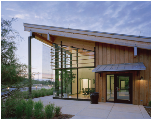
Figure 4-20. Glass-terraced wall with shading.
