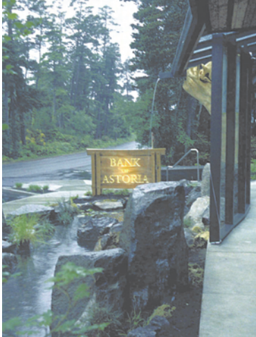
Figure 3-14. Water from the roof is discharged through a scupper into a landscaping pond for storage and settling before the water is reabsorbed into sandfill below.
