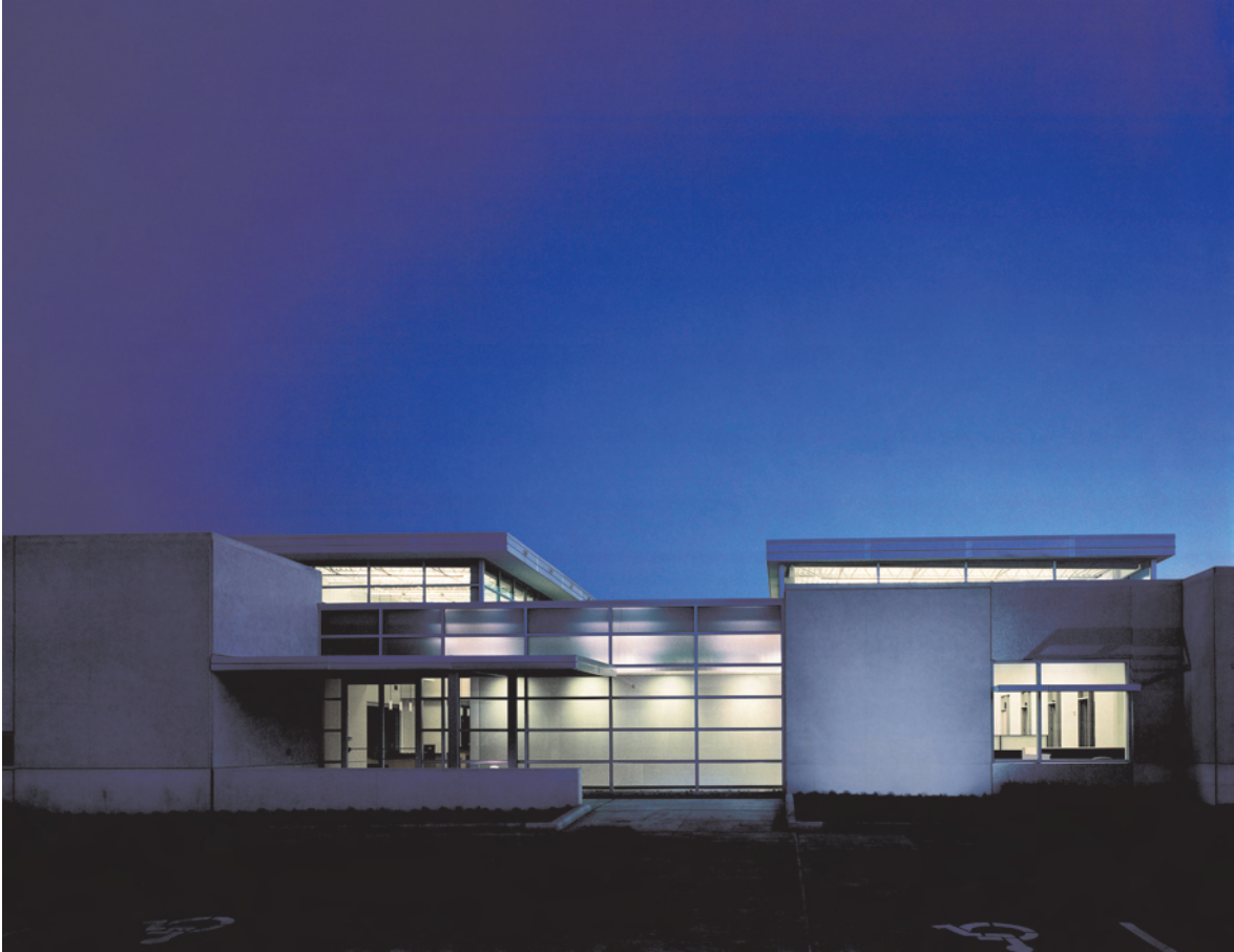
Figure 3-6. SpawGlass Construction Corporate Headquarters is calculated to be 56 percent more efficient than the baseline standard due to building orientation, window protection, a light-colored roof, and electrical and HVAC choices.
