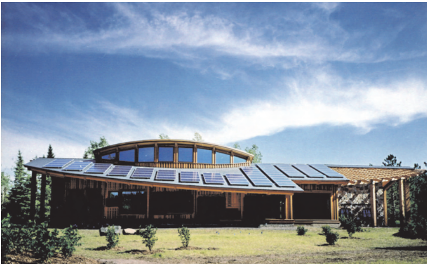
Figure 3-26. The Hartley Nature Center was built on a south-facing slope, which has provided the center great exposure to sunlight.
