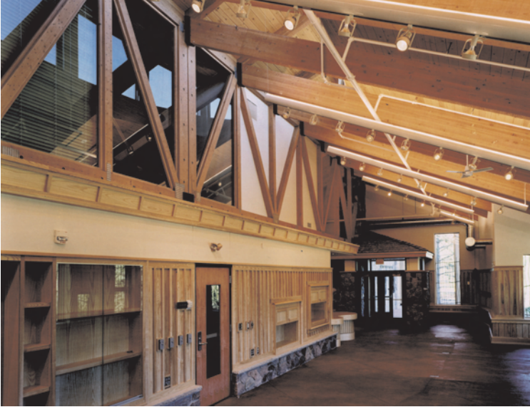
Figure 3-25. The center features such sustainable and environmentally preferable building materials as 100 percent recycled content roof shingles, recycled content ceiling tiles, and FSC-certified wood.
