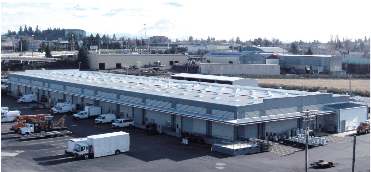
Figure 4-1. Tacoma Power & Light new shops building featuring an array of skylights for interior daylighting.
