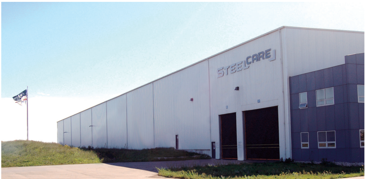
Figure 4-3. Exterior view of Steelcare, Inc.
