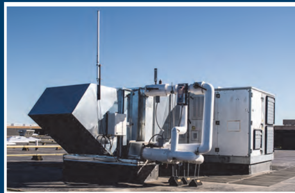
Delivery of Glycol to AHU
