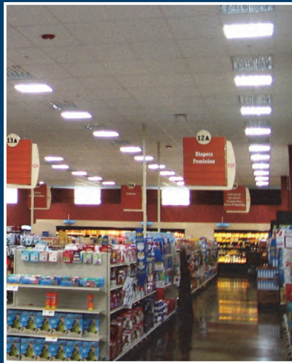
Tubular Daylighting Device Diffusers on the Grocery Sales Floor Photographs reproduced with permission of Giant Eagle, Inc.
