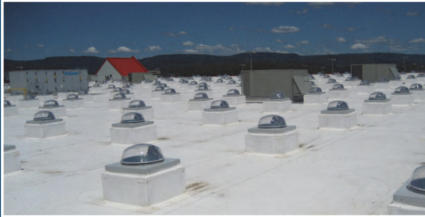
Roof-Mounted Domes for Tubular Daylighting Devices
