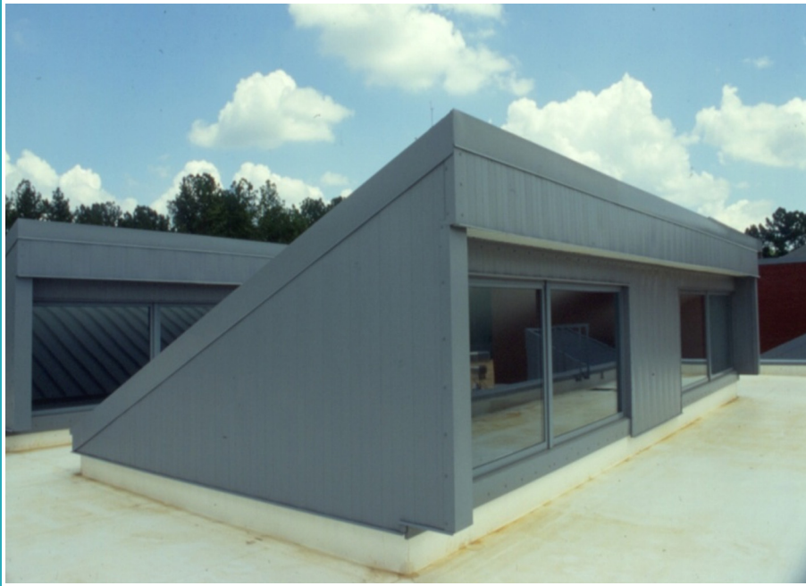
South-Facing Roof Monitor
