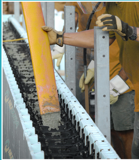
Construction of an Insulated Concrete Form Wall
