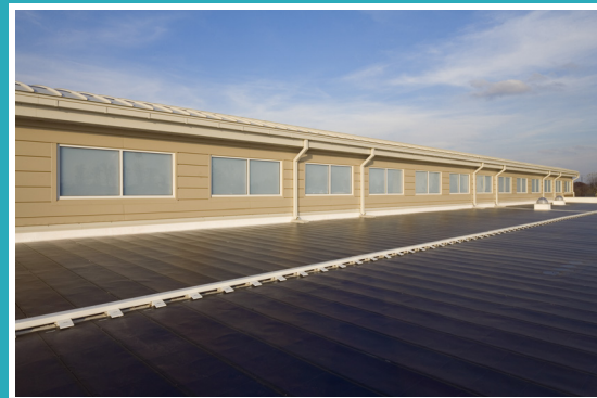
(Left) Daylighted Classroom and (Right) Rooftop Thin Film and Crystalline PV Panels Source: Rachel Paul Photography (for CMTA Engineers)
