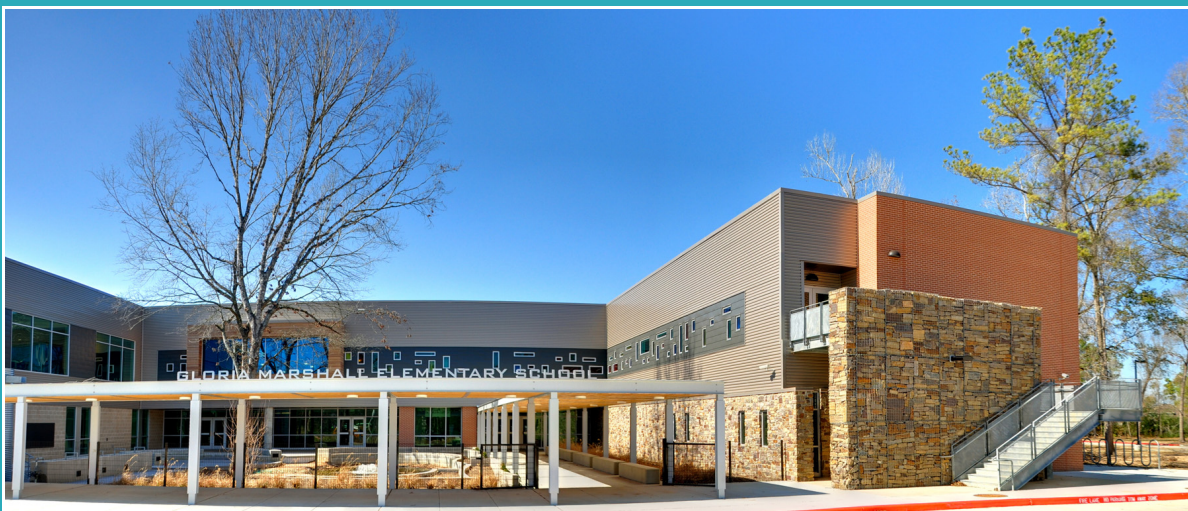
Gloria Marshall Elementary School Exterior Source: SHW Group
