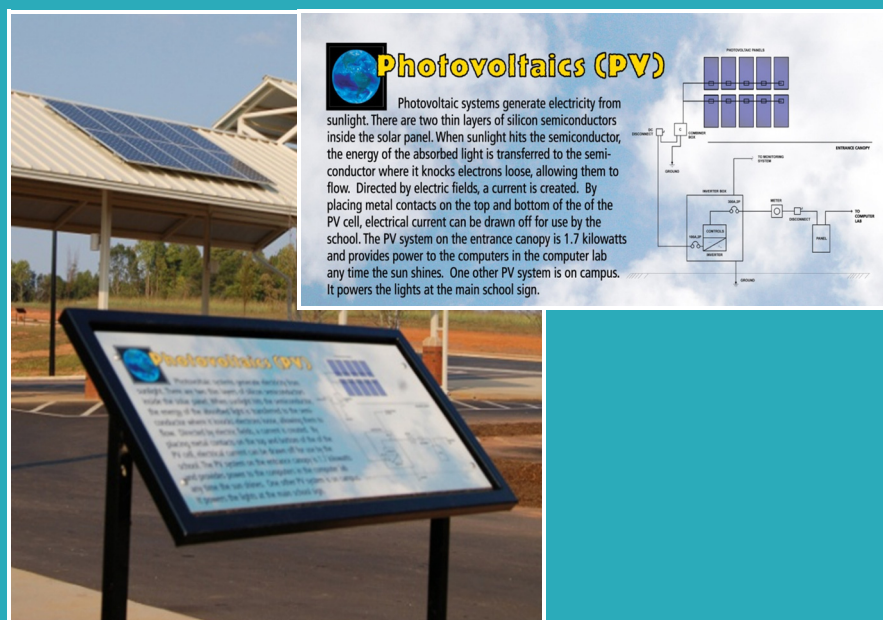
Photovoltaic System with Information Sign
