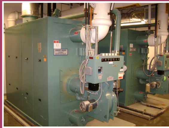
Campus 1: Domestic Water Heaters (left) and High-Efficiency Water Tube Boilers (right)
