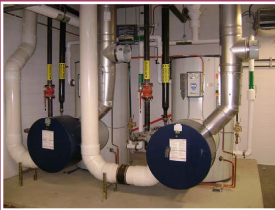
Campus 1: Domestic Water Heaters (left) and High-Efficiency Water Tube Boilers (right)
