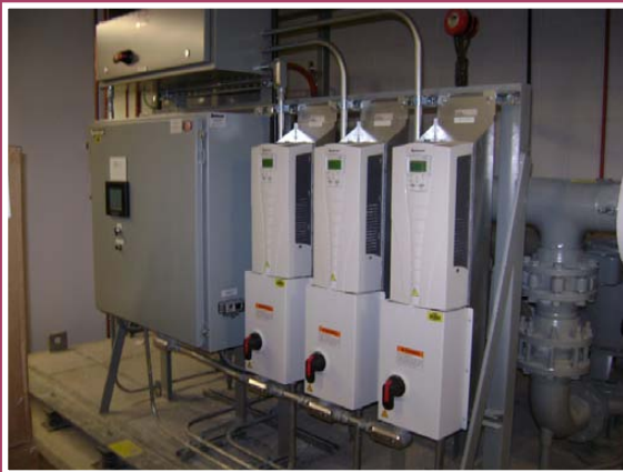
Campus 1: Pumps with Variable Frequency Drives (VFD) (left) and Emergency Generators (right)
