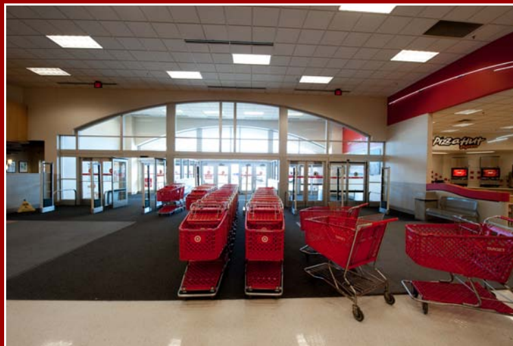
Target Vestibule Design with Clerestory Glass Photography courtesy of NREL; Credit: Dennis Schroeder
