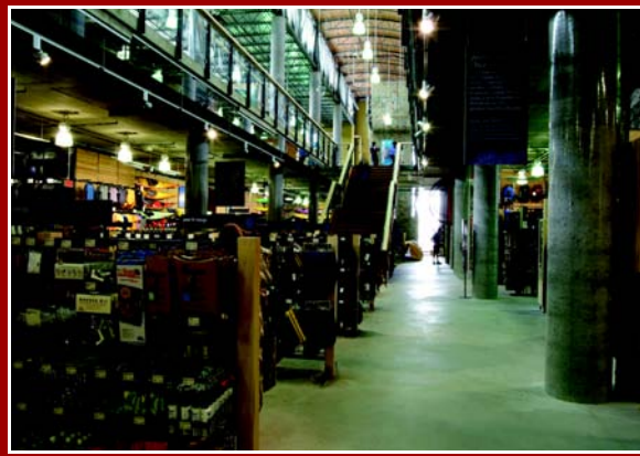
Bare Concrete Floors with Protective Coating
