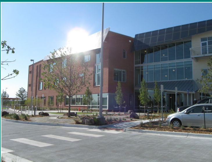
Main Entry on South Face
