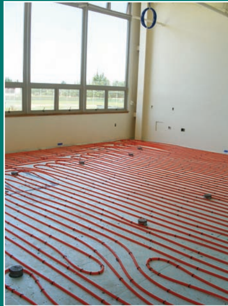
PEX Tubing in Serpentine Pattern
