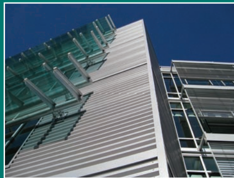
Exterior Tinted-Glass Shades Used on the East and West Façades†
